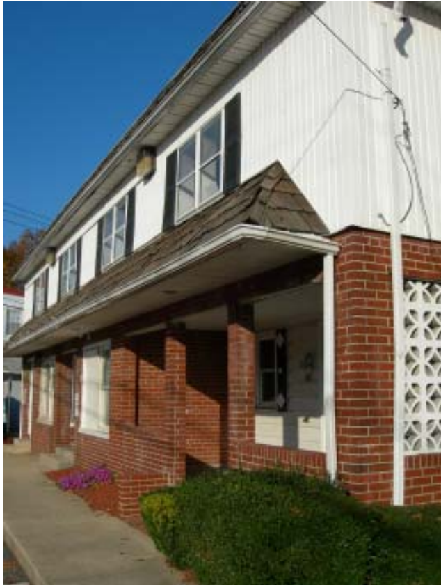
Detail of building at left (MBA)
