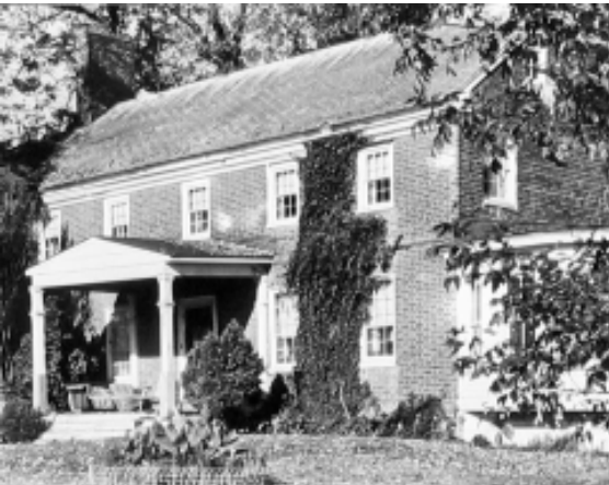
Front View with porch intact
