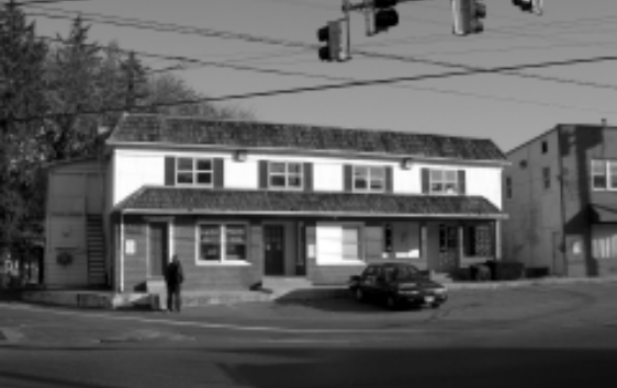
Mixed-use building, Sandy Spring MBA
