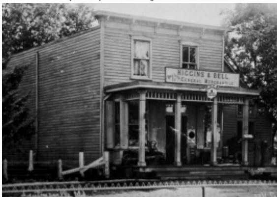
General Store, Laytonsville (demo) SSM
