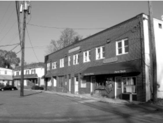
Mixed-use building, Sandy Spring MBA
