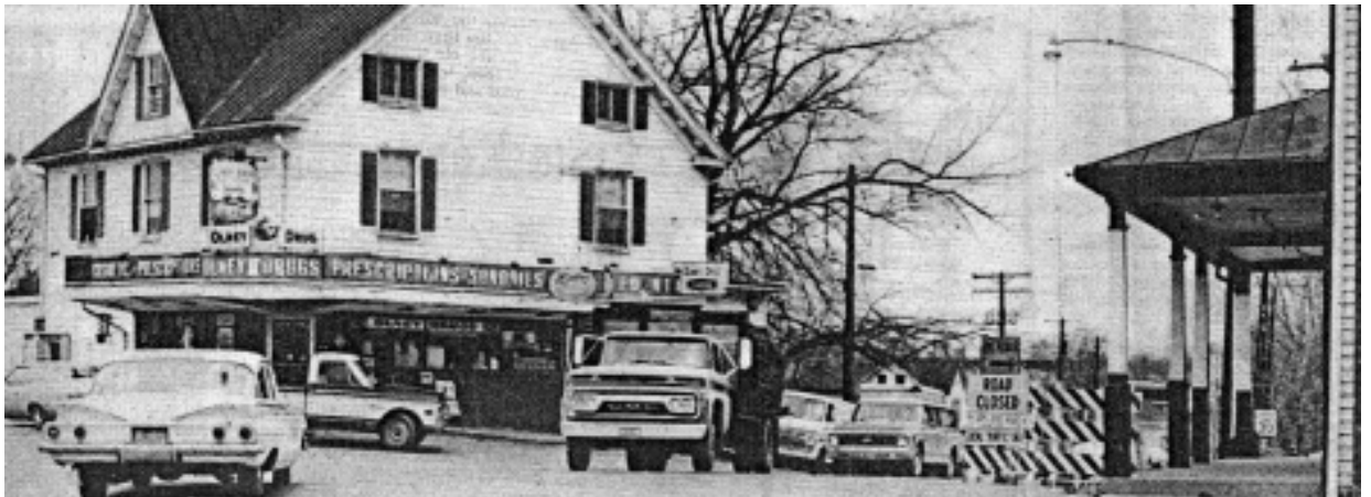
View north on Georgia Avenue, circa 1977 (SSM)
