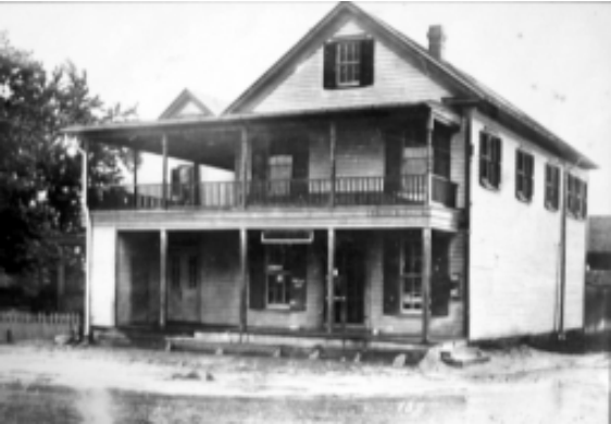
Stone St. Store, Laytonsville (demo) SSM
